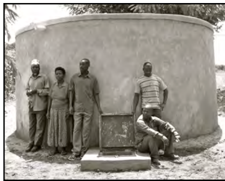
We now will be able to collect rainwater that runs off the school roof and store it in the cistern!
