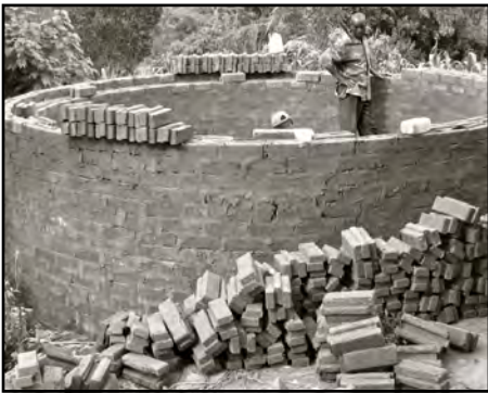
The 40,000-liter rainwater cistern being built.
