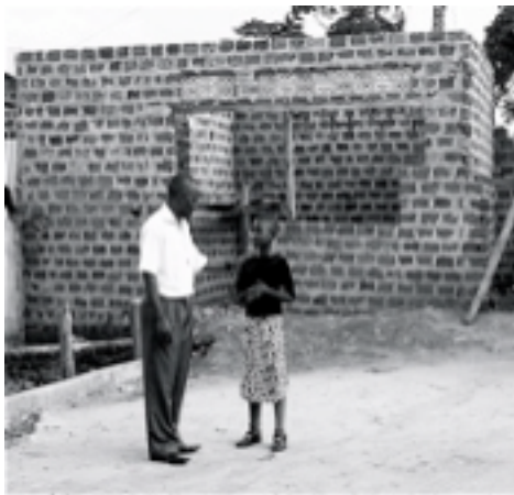
New (in progress) brick kitchen
